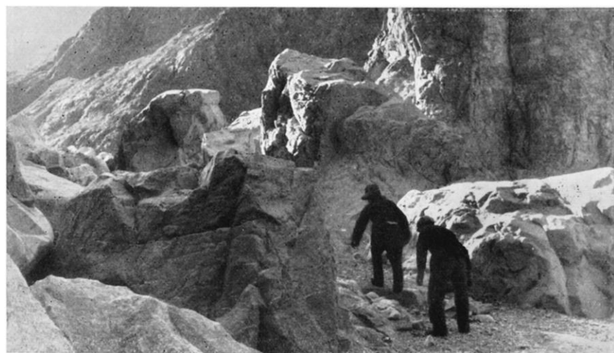
Working on the road in the Toksun gorge
